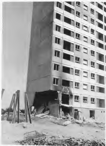
Plate No 9 A block in Algeria, damaged by an explosion
